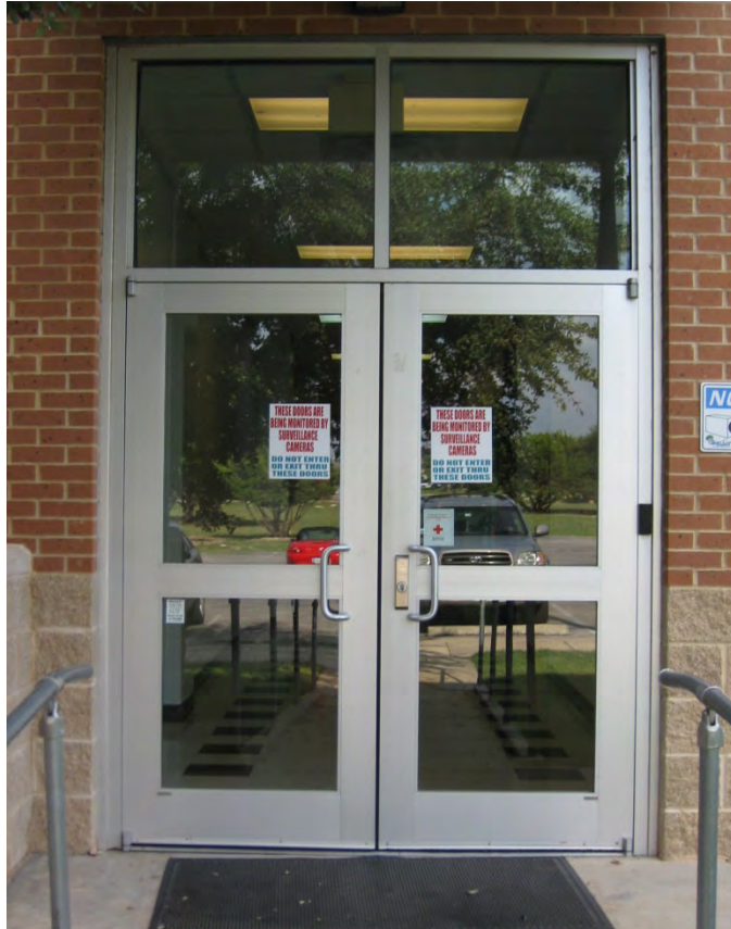
Image of aluminum storefront system at west exit
