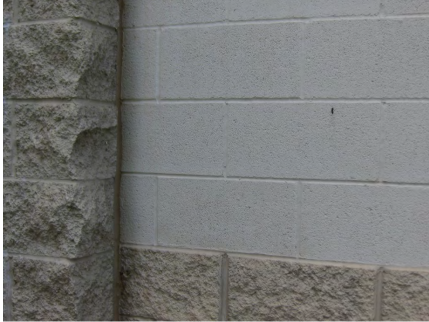
Example of single wythe Concrete Masonry Units (CMU) with elastomeric coating
