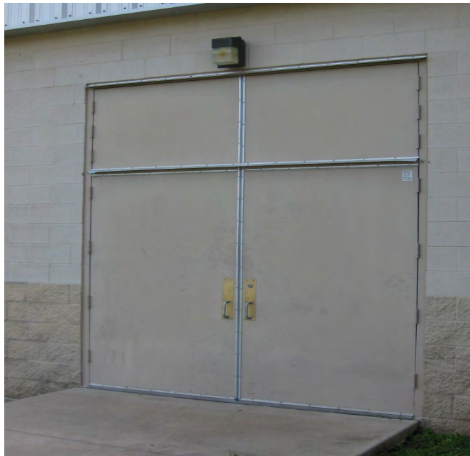
Image of painted hollow metal doors at gymnasium
