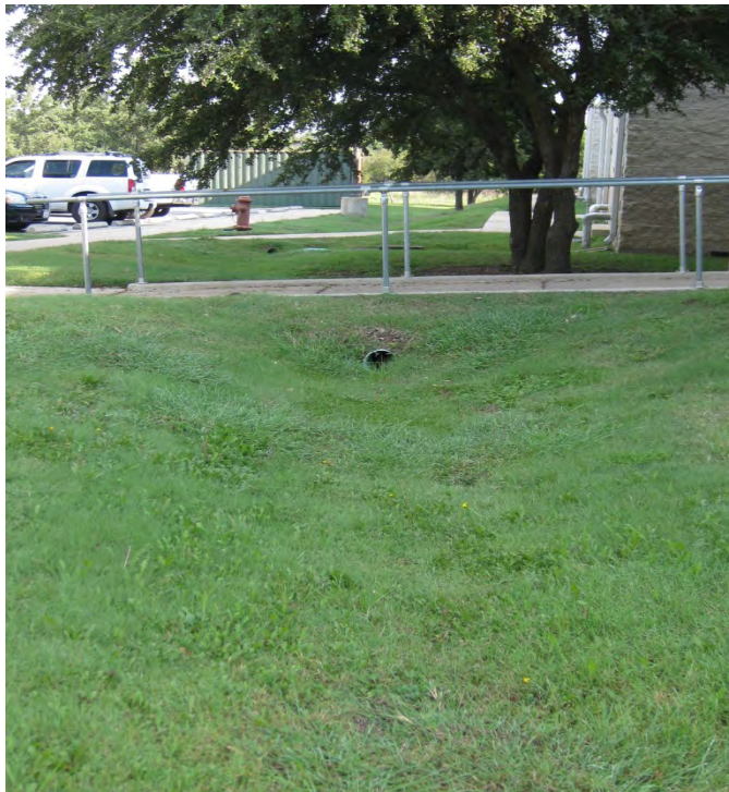
Image of drainage swale as it continues around the west side of building
