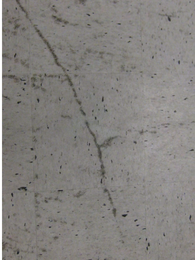
Image depicting poor condition of vinyl composition tile at game room
