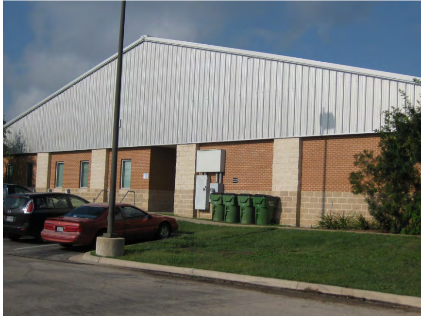
Example of Concrete Masonry Units (CMU), brick and metal wall panels
