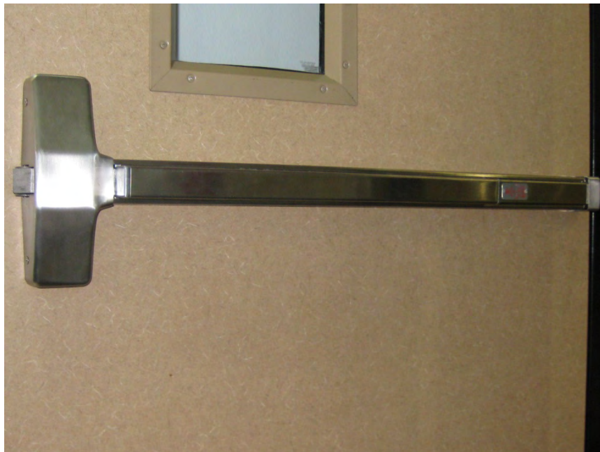
Typical good condition of door hardware within the building
