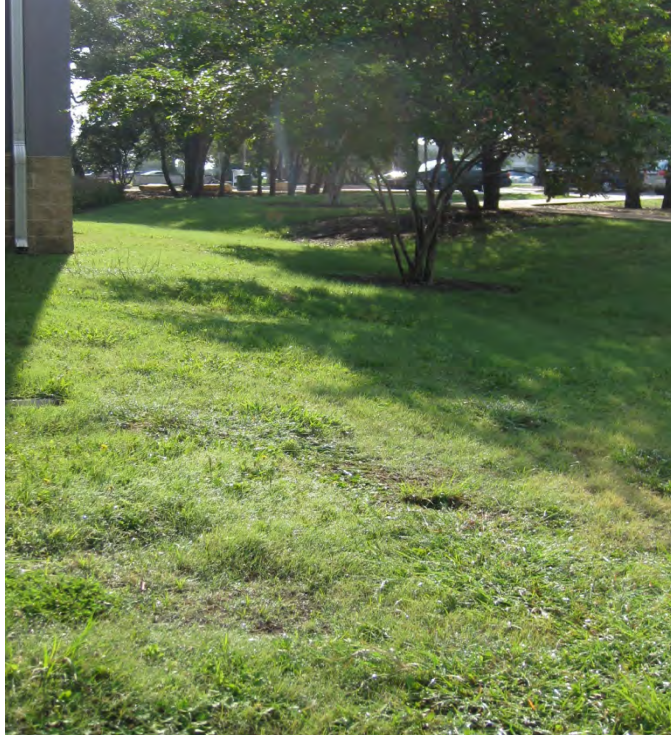
Image of drainage swale at front (south) side of building
