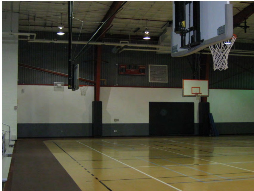
Image of overall condition of gymnasium floor
