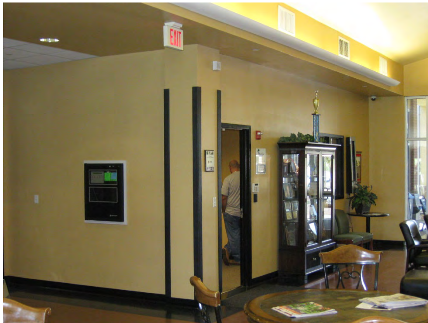
Interior gypsum wallboard at main lobby
