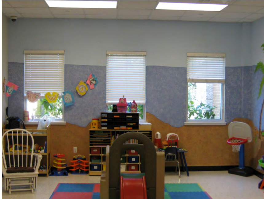
Interior gypsum wallboard at children's area
