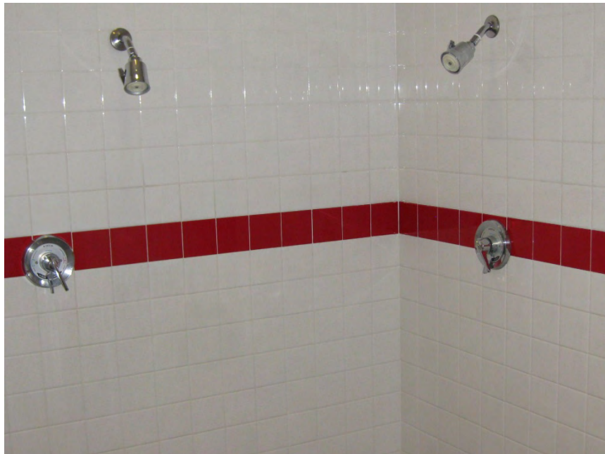
Interior ceramic wall tile at men's showers
