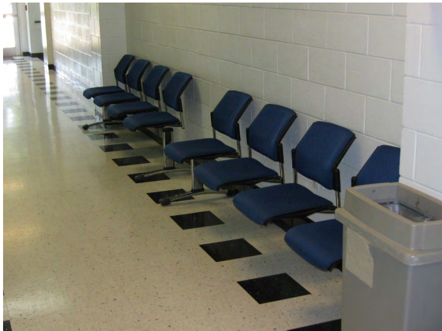
Interior painted concrete masonry units (CMU) at west corridor
