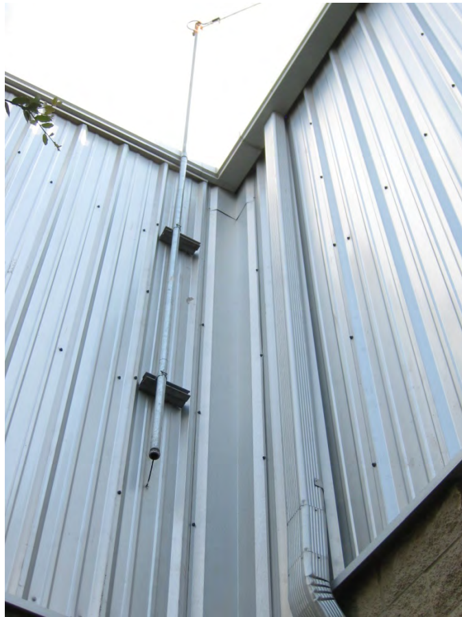
Example of metal wall panels
