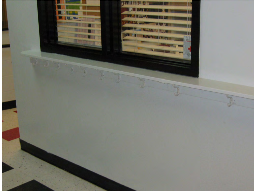
Interior painted gypsum wallboard at west corridor
