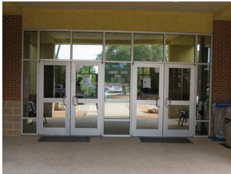
Image of aluminum storefront system at main entrance
