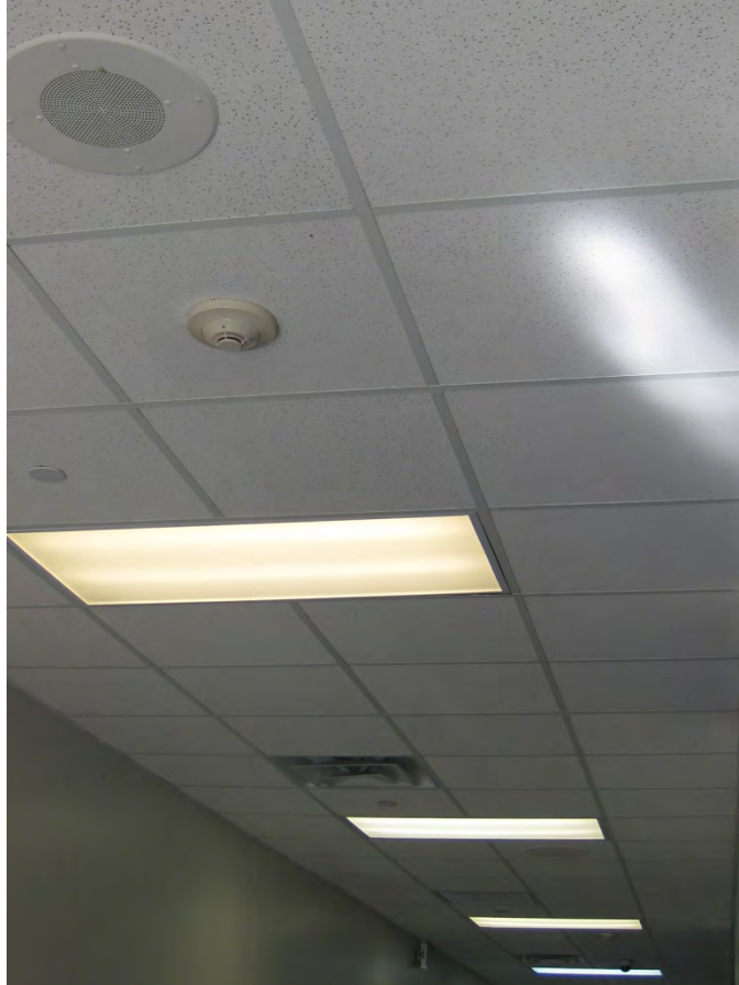
Typical good condition of ceilings at the facility
