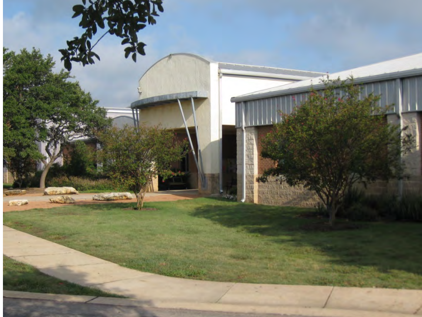
Example of Concrete Masonry Units (CMU), brick, plaster and metal wall panels
