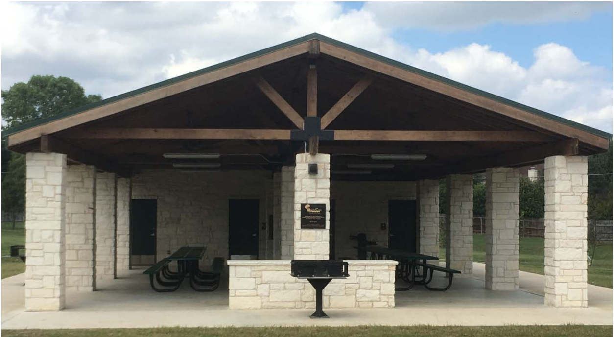
Cat Hollow Park Pavilion - Completed March 2016
